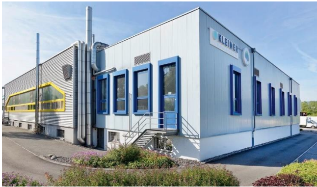
O. KLEINER AG production facility
